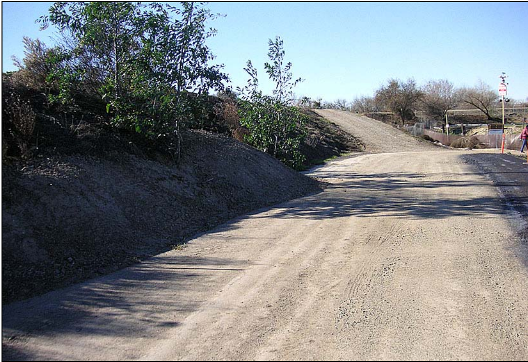
Source: Photograph taken by Reclamation District No. 17 in 2009 Image A: Reach VIIf—Looking West
