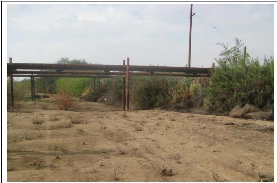
Photo 6B: Picture of Focus Area 4 (Kern River Crossing) taken on 11/1/2010, facing southwest. All construction activities would occur within a 20-foot corridor along the east side of the existing pipe bridge (pictured in the foreground).
