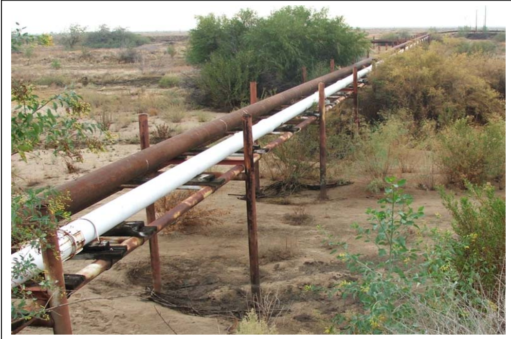
Photo 6A: Picture of Focus Area 4 (Kern River Crossing) taken on 10/18/2010, facing southeast. The existing 16" pipeline (pictured on the left) crosses the Kern River, above-grade on existing support structures (a pipe bridge). The crossing length over the Kern River is approximately 641 feet.
