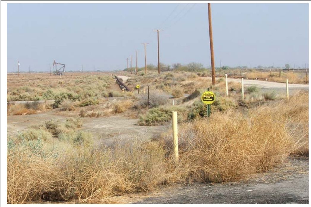
Photo 5A: Picture of Focus Area 3 (Pipeline segment that parallels the Kern River) taken on 10/18/2010, facing north-northeast. The existing 16" pipeline is positioned approximately 25 feet north of the levee toe (approximately 75 feet from the Kern River) and runs parallel to the Kern River, above grade, on existing support structures within the ROW.
