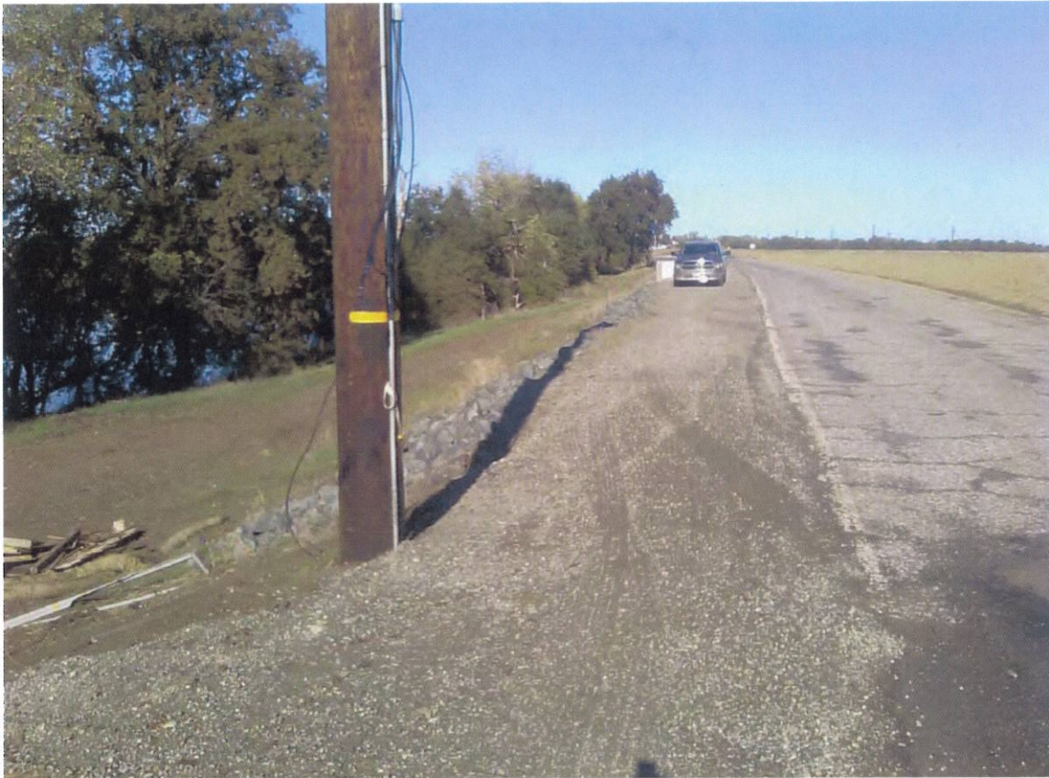
Photograph 1. Looking north along Garden Highway at electrical service pole at Cummings Pumping Plant.
