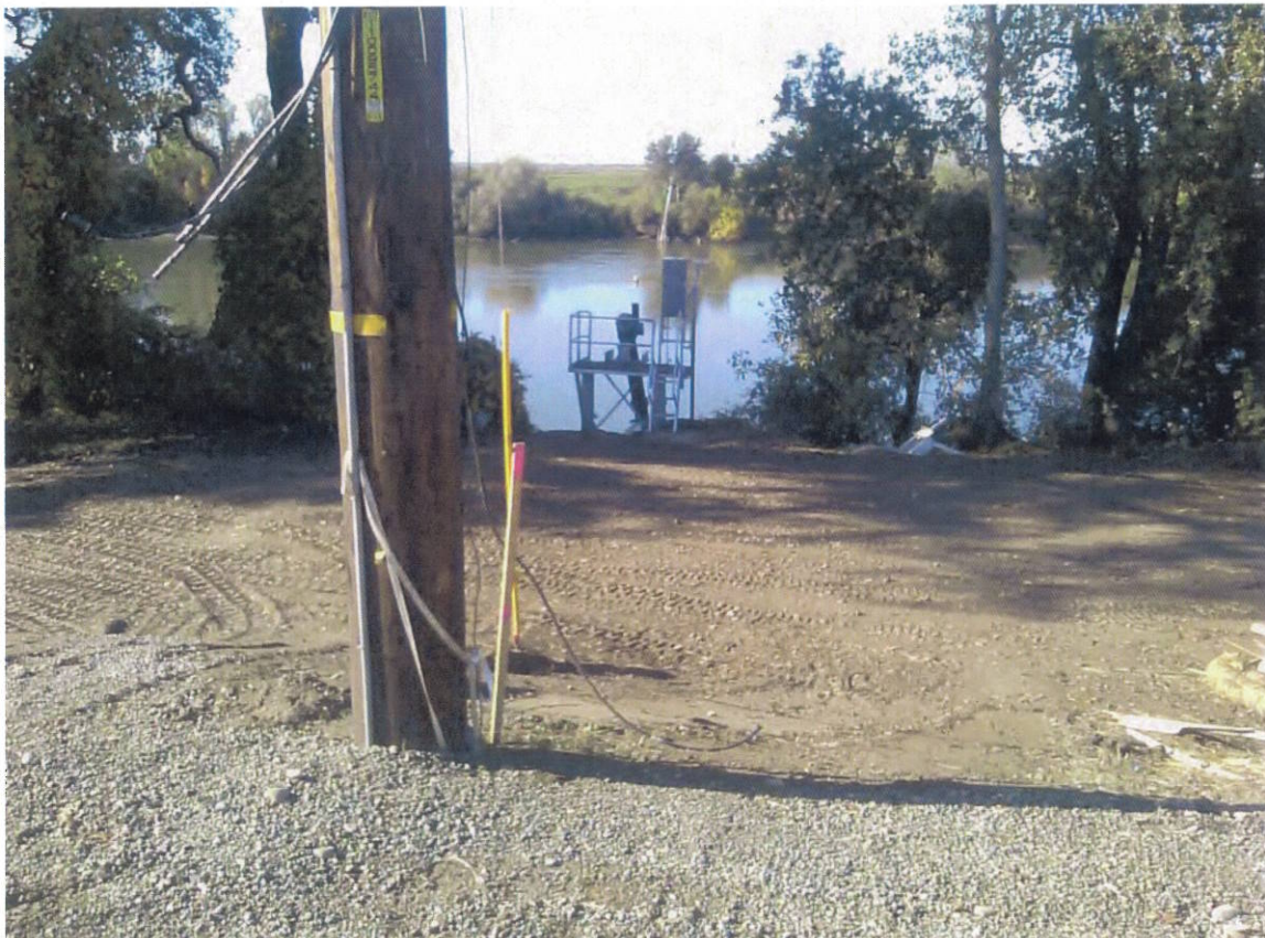
Photograph 2. Looking west from Garden Highway towards Cummings Pumping Plant and Sacramento River.
