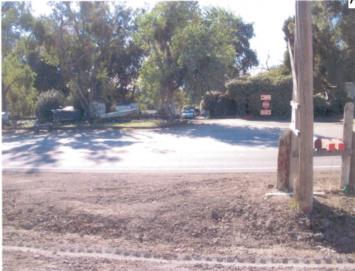
Photograph 1. Looking west at proposed pipe crossing location across Sacramento River East Levee towards Verona Village Resort and Marina.
