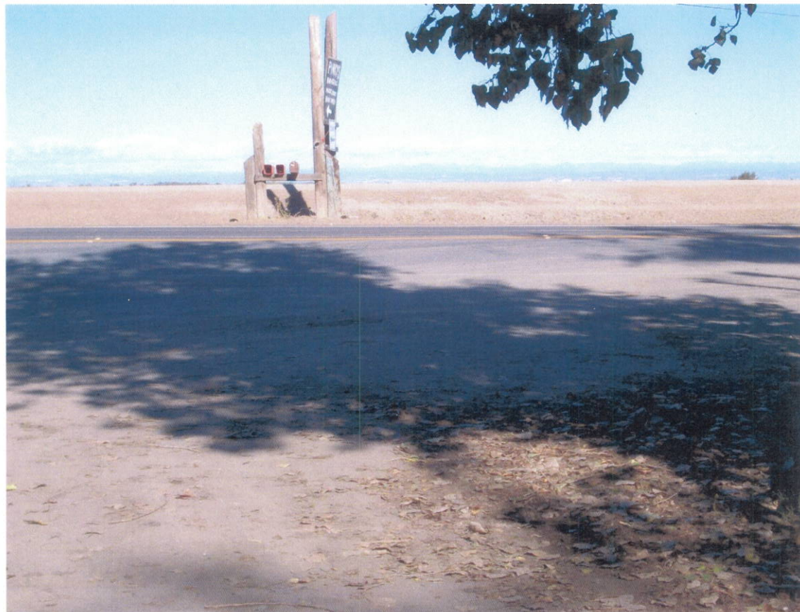
Photograph 2. Looking east across Garden Highway and Sacramento River East Levee at location of proposed pipe crossing.
