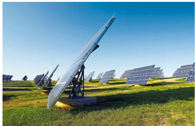
Photo 3.1: Dual axis solar tracker
