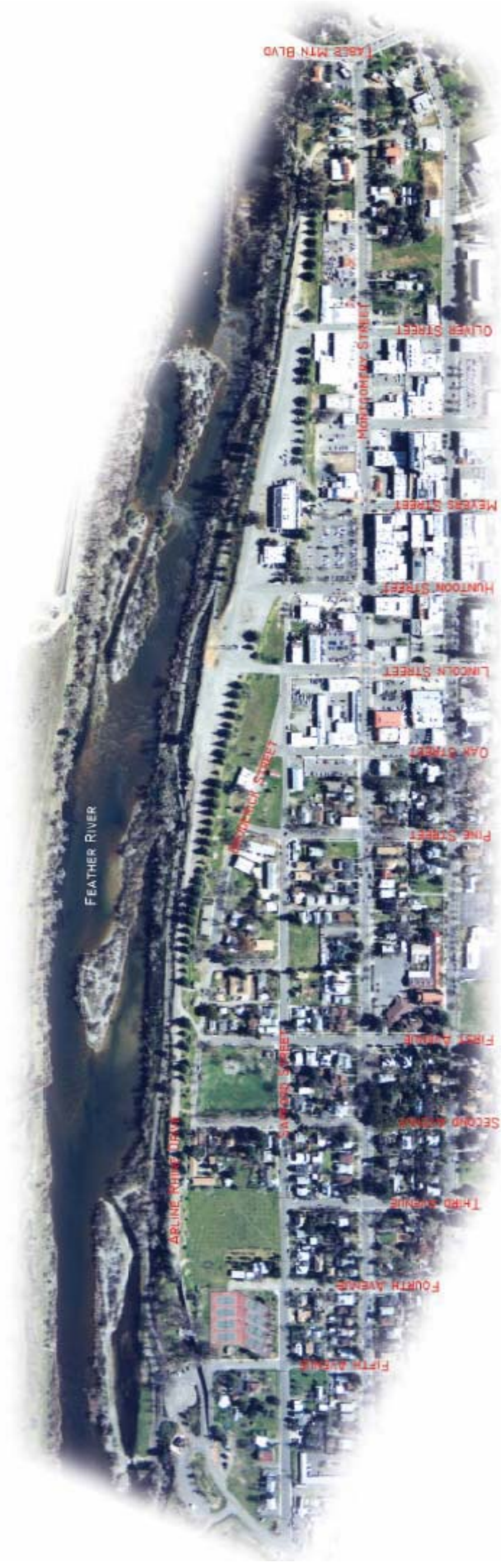
Figure 2 Aerial Photograph of Project Site
