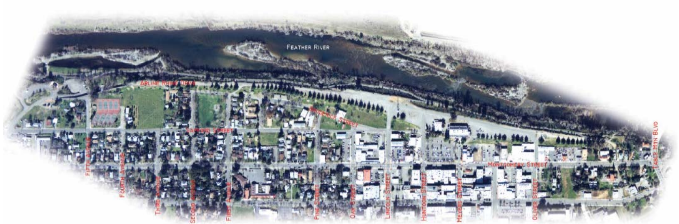
Figure 2 Aerial Photograph of Project Site
