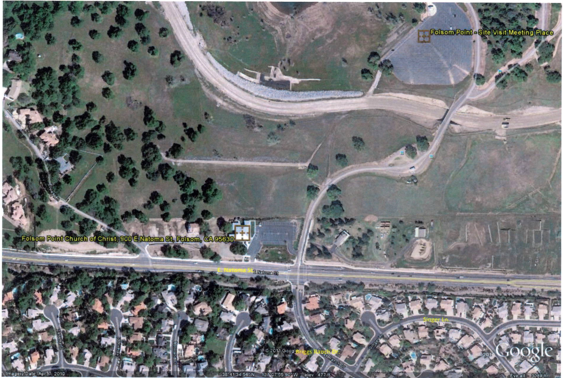
An aerial view of Folsom Point and adjacent roads.
