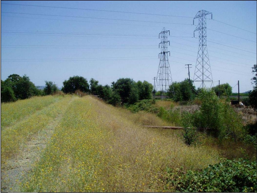
Honcut Creek Levee, looking east at tower 13/99.
