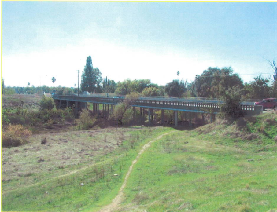
Photo 3: Looking downstream from north levee
