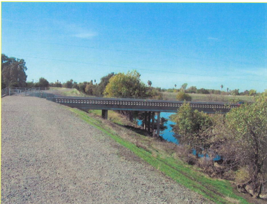
Photo 4: Looking downstream from south levee
