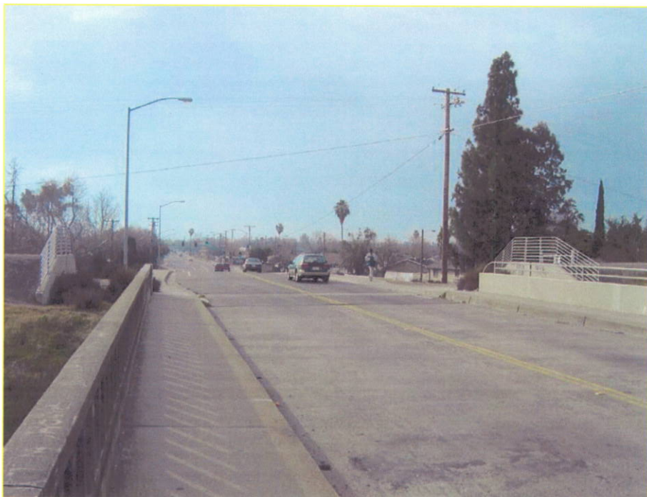
Photo 2: Looking south from bridge sidewalk
