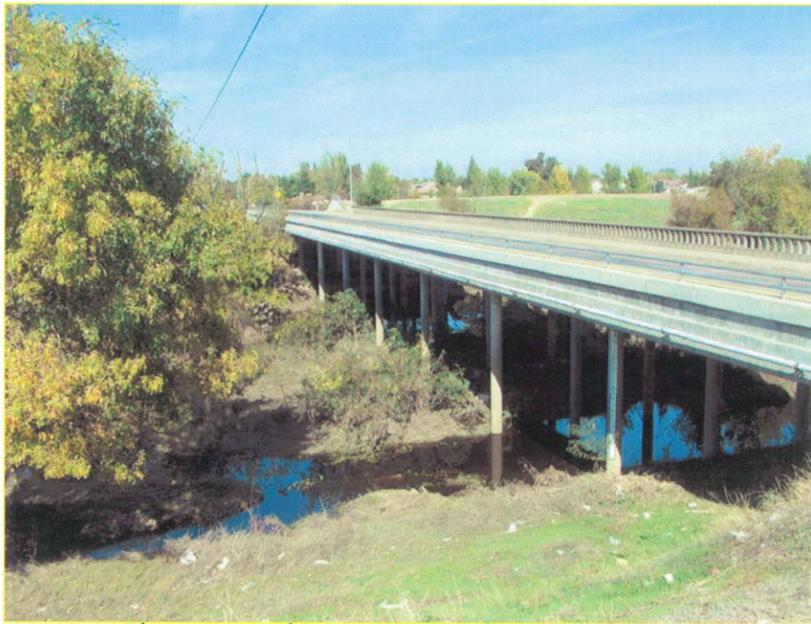
Photo 1: Looking upstream from south levee
