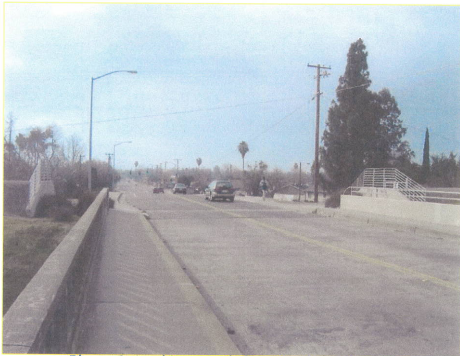
Photo 2: Looking south from bridge sidewalk
