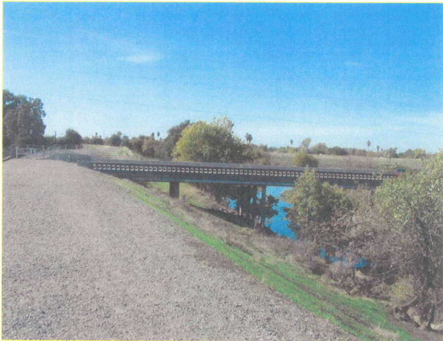
Photo 4: Looking downstream from south levee
