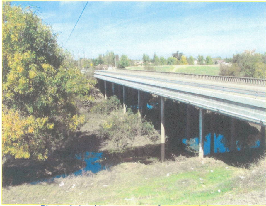
Photo 1: Looking upstream from south levee
