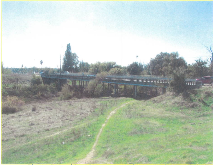
Photo 3: Looking downstream from north levee
