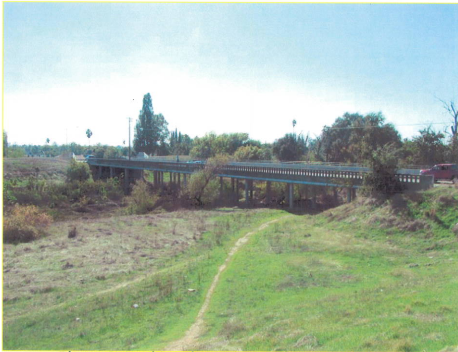
Photo 3: Looking downstream from north levee
