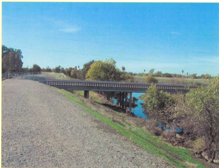
Photo 4: Looking downstream from south levee
