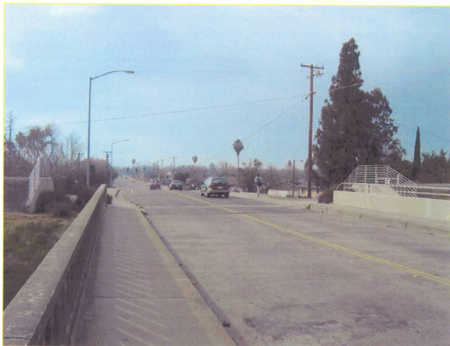
Photo 2: Looking south from bridge sidewalk
