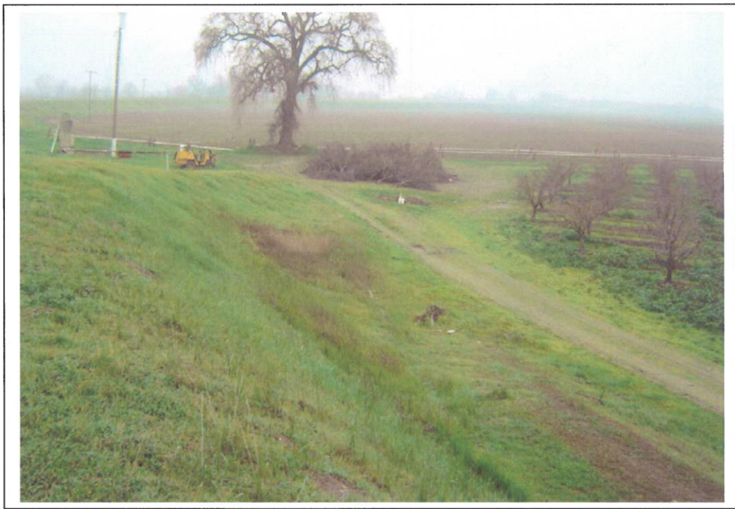
View of landside looking upstream.
