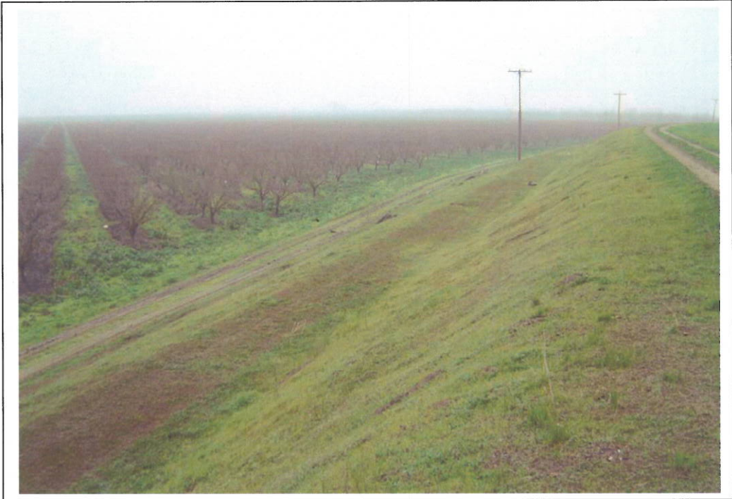
View of landside looking downstream.
