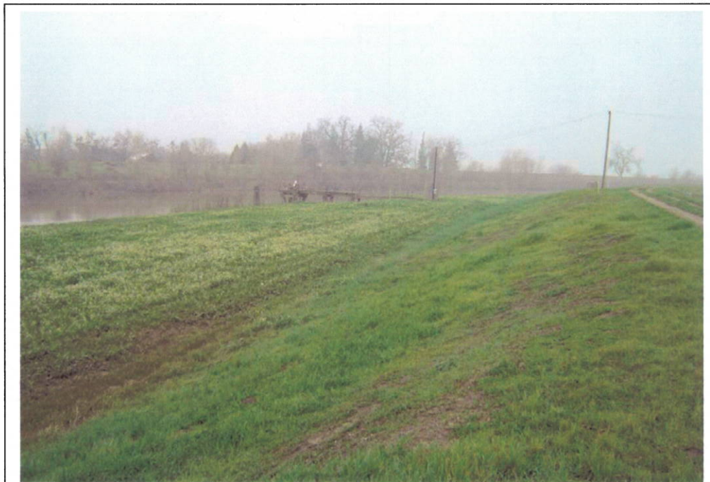
View of landside looking upstream.
