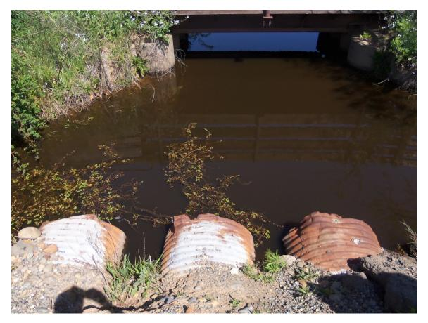
Looking North at Elder Creek where it crosses Elder Creek Road of the existing three 36" Corrugated Metal Pipe (CMP) culverts.
