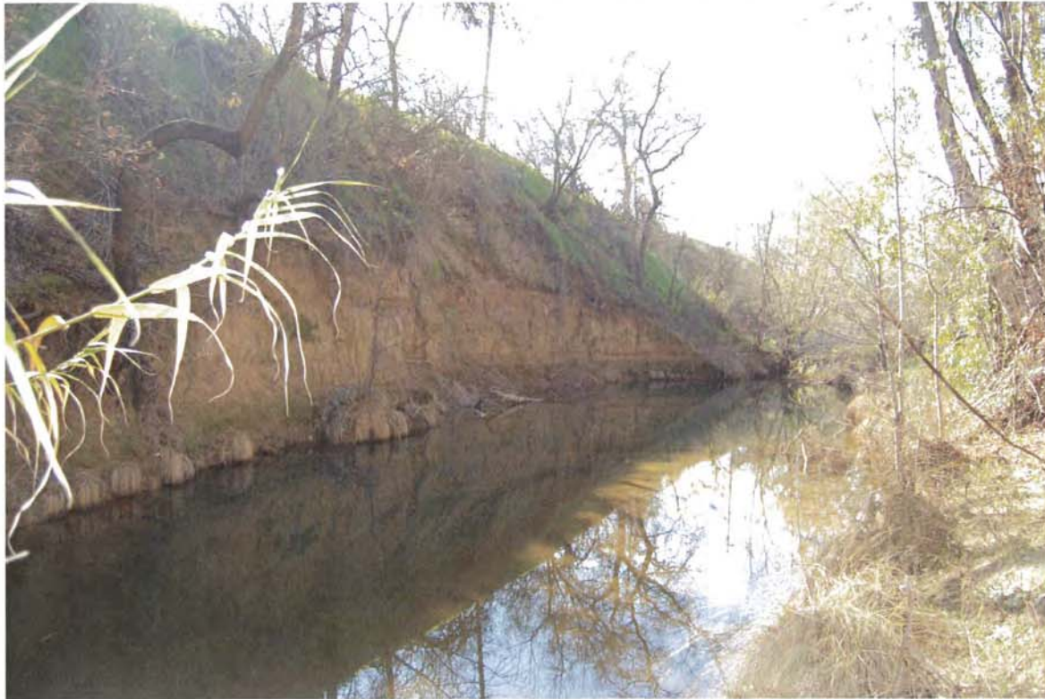
Photo 2 – Looking southwest at bank erosion shown in Photo 1. This is the southern branch of low-flow channel that will be filled during Phase 1.
