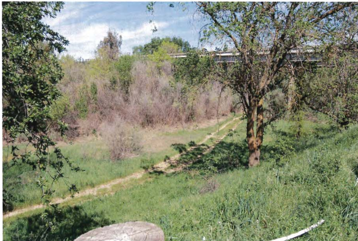
Photo 4 – Looking northeast at the south side floodplain and the I-505 bridge. A side channel with spawning gravel will be installed in this area of the floodplain during Phase 1.
