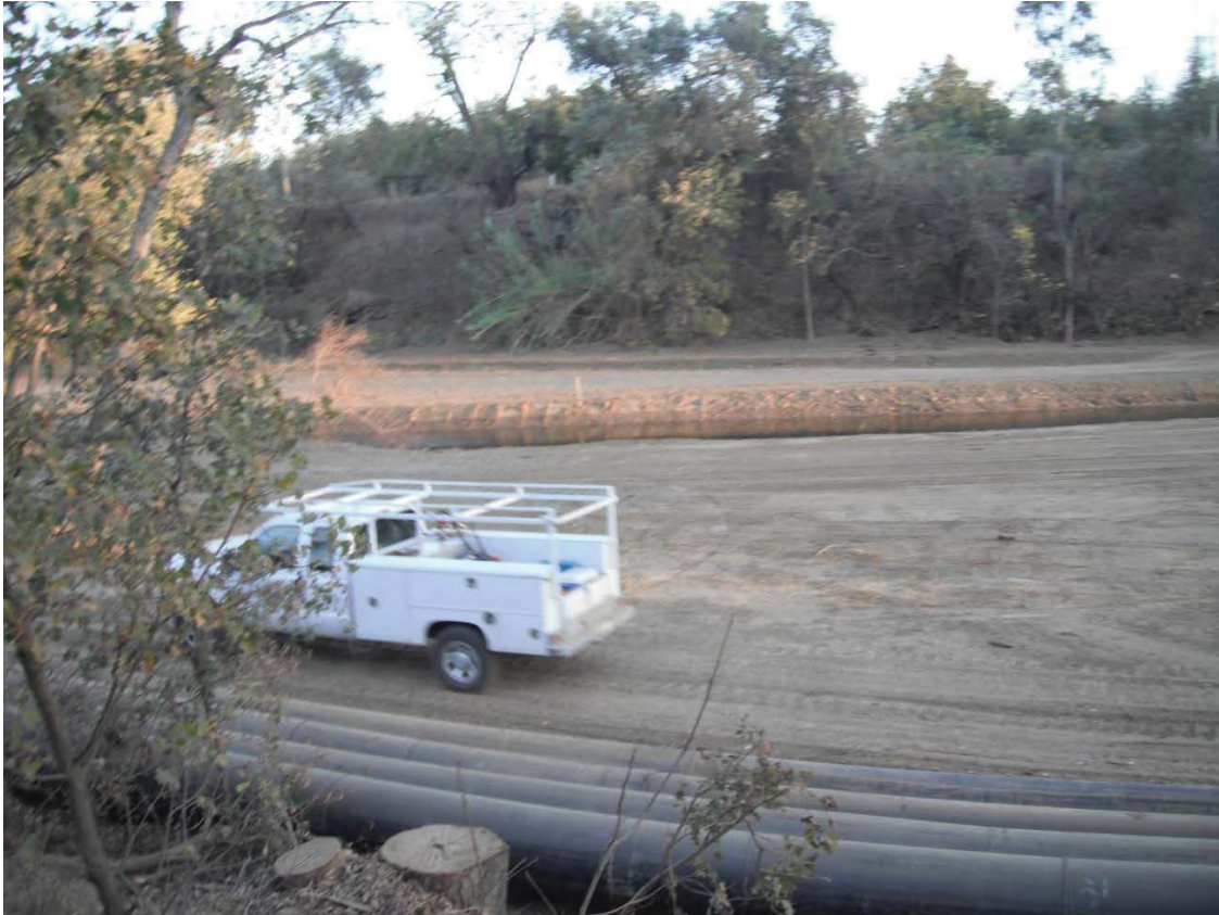
Figure 1: As built floodplain in Phase 1
